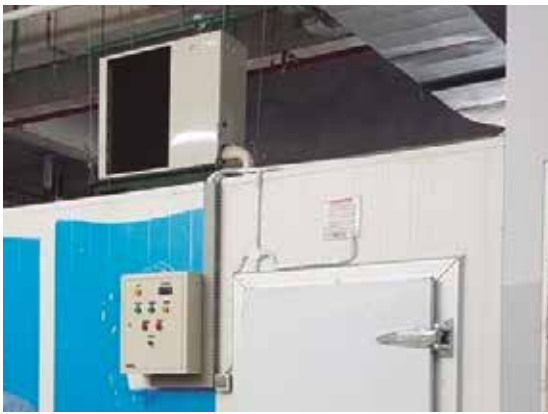
Picture of the PAC 3 Tecumseh condenser unit installed and front view.
